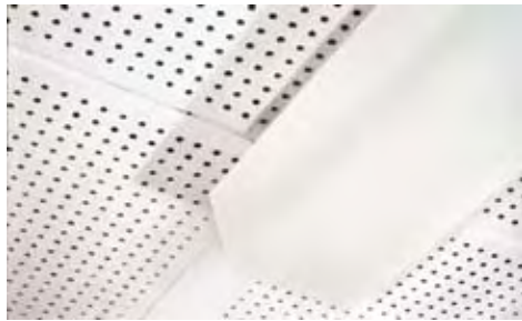
Perforated AIB ceiling tiles
