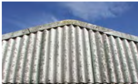
Asbestos cement wall cladding
