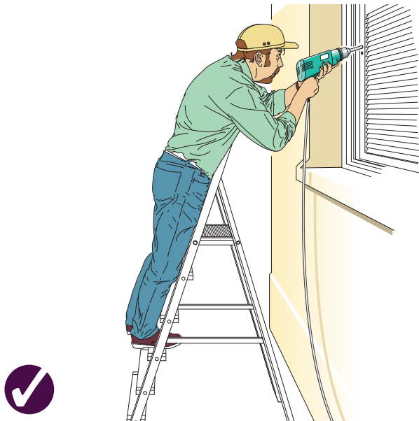
Figure 3a Correct - rungs facing work activity
